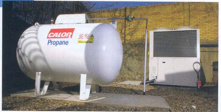
Sanyo's LPG-driven air-conditioning concept provides a solution on sites with restricted electricity supply and no mains gas.
